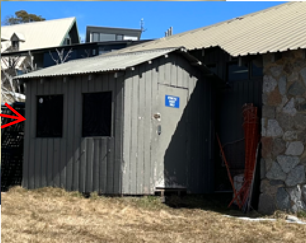
Existing temporary shed to be removed to facilitate development
